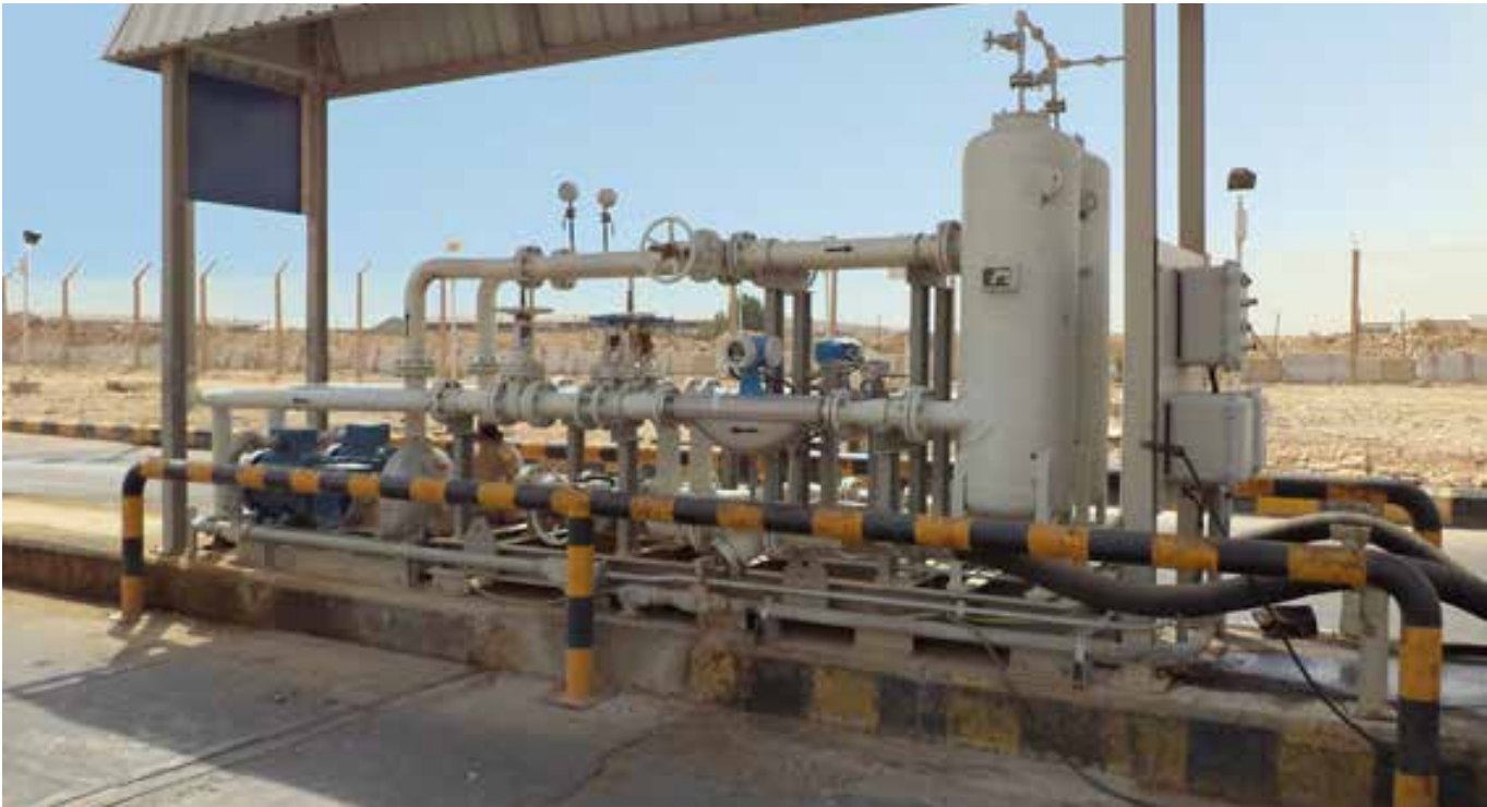
Truck loading system, Saudi Arabia
